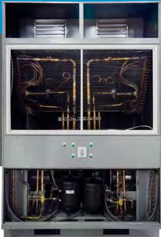
Front View (From inside the conditioned area). Note redundant piping for dual refrigeration circuits including two receivers
